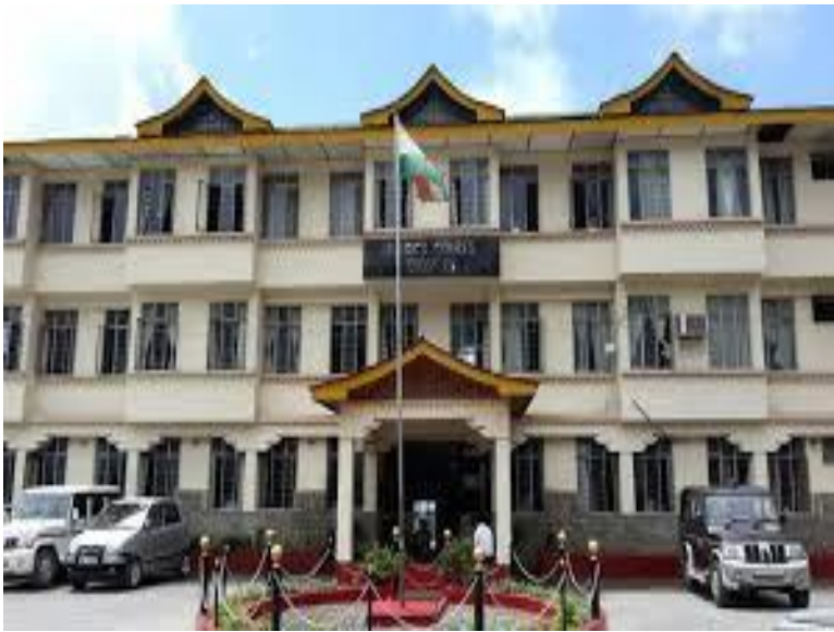
District Courts Complex Namchi, South Sikkim
